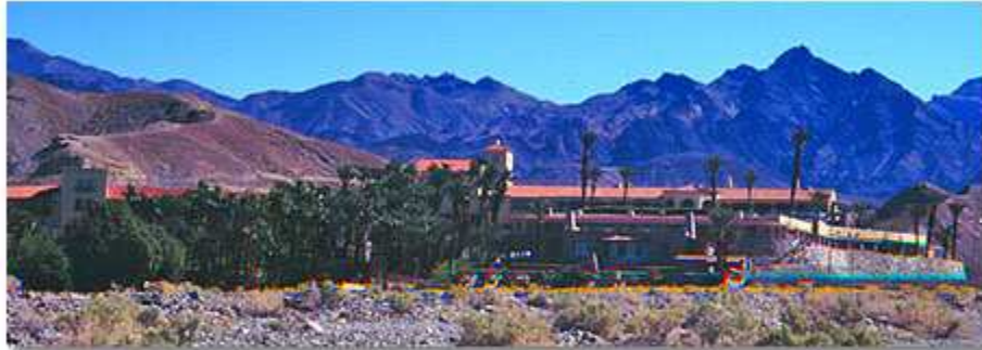
The Furnace Creek Inn was originally built to accommodate borax company officials who came to Death Valley to check on operations. It later became a luxury resort.
